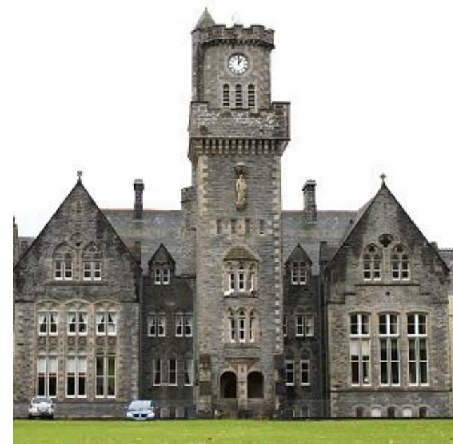
The Highland Club (former Abbey + Fort) from the canal towpath
